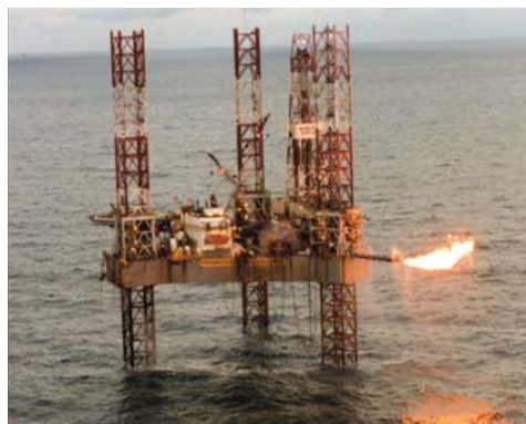
47/10-7y Helvellyn Well being tested at 60 mmcsd
